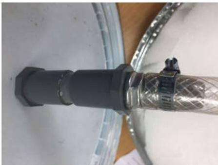
**Figure 5a: The connection between container cap and drainage pipe**
